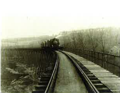
Foto 13: Viaduct over Gulpdal in 1925 (bovenaanzicht)
