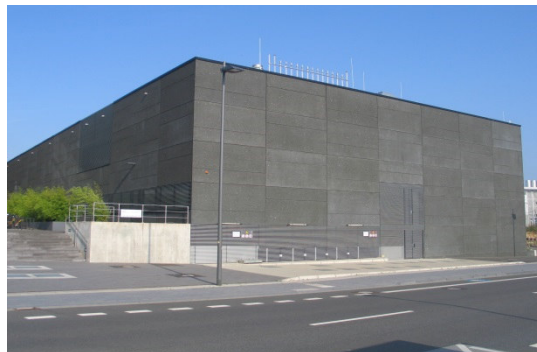
CMP Center for mobile Propulsion
